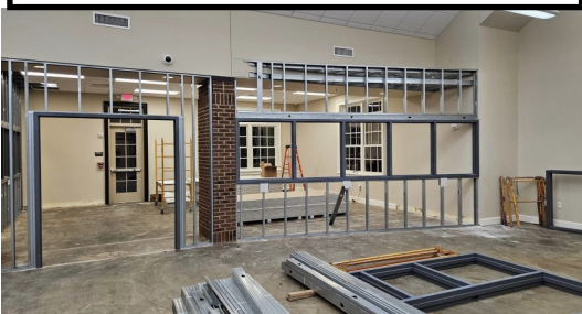
Maker Space walls and door frames are up!
